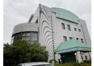
Prefectural HS Mie Dream Academy Training Building (Proposed Location for the Junior High Night School)
