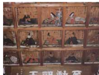
Latticed pattern ceiling of Daisho-ji
