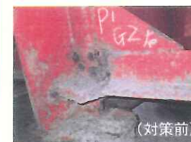
橋梁修繕状況
