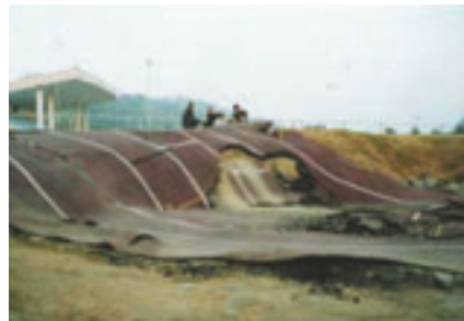
The reverse fault caused by the Taiwan Shushu Earthquake (M7.7) in 1999. (2 meter vertical ground slippage occurred at this primary play ground)
