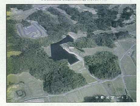
大谷池調整池 Otanlike Regulating Reservoir
